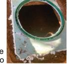
a plastic riser system. Concrete septic/well covers can be heavy and hard to lift in-order to gain access. Concrete covers also begin to degrade over time and fall apart. Converting these concrete septic/well covers with a plastic riser system makes a safe and easy way to gain access to your home's critical water and septic components.
